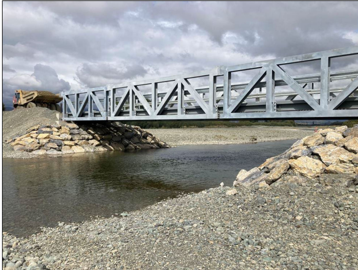
Temporary bridge in place during extraction.
