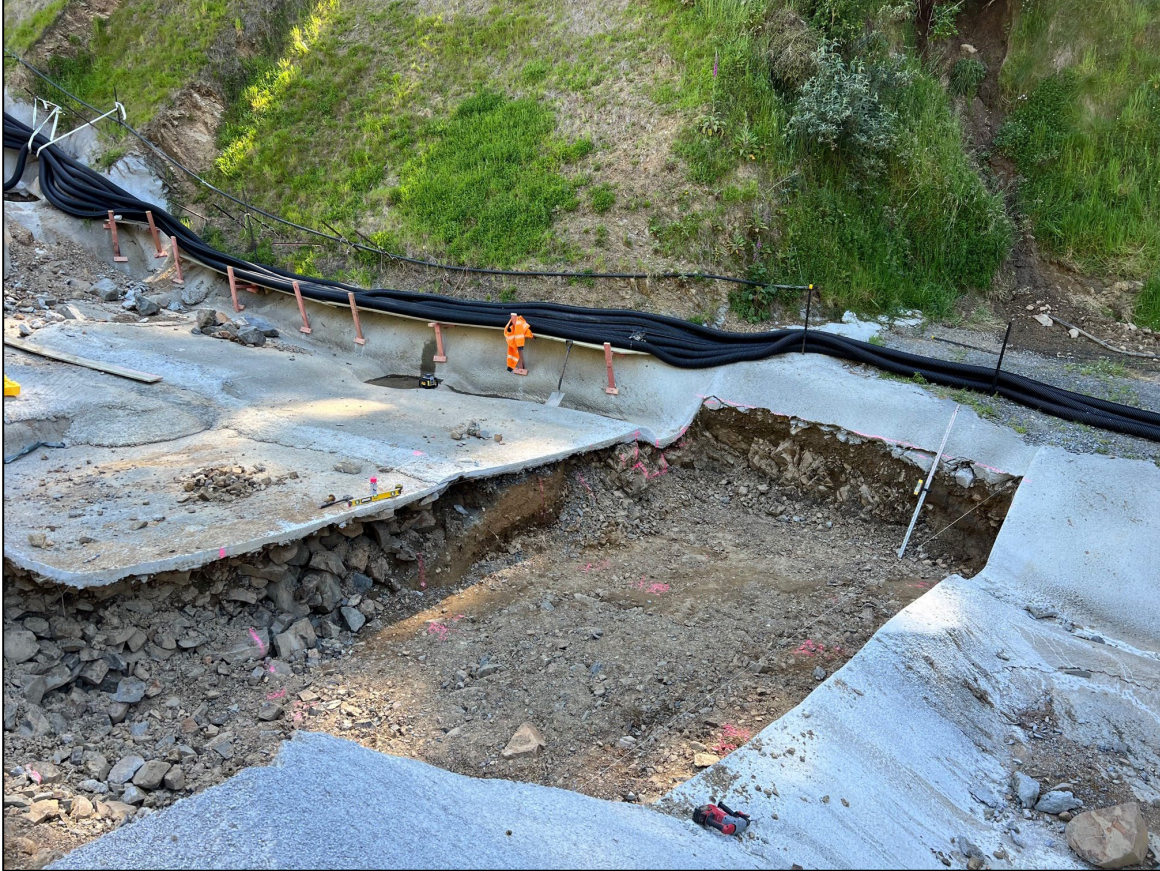
Drift deck installation.
