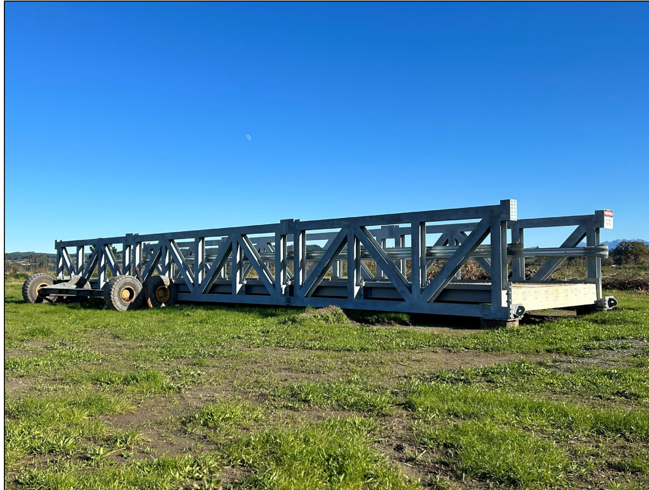
Bailey bridge used to cross the river when extracting.
