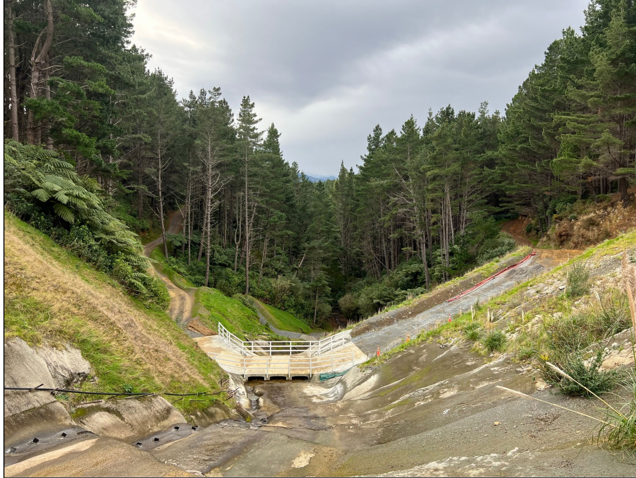
Drift deck for access and water flow.
