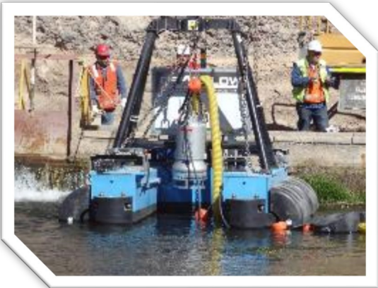
Remotely operated dredge, cable mounted
