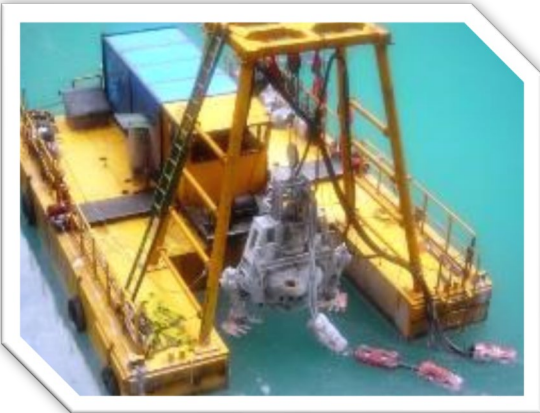
Manned dredge, cable mounted
