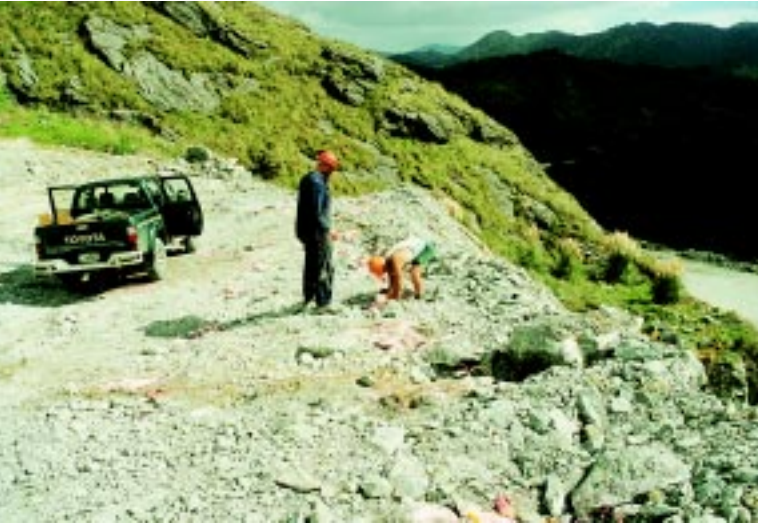
SETTING BLASTING EXPLOSIVES
