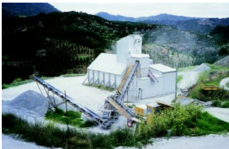
TYPICAL LIME PLANT
