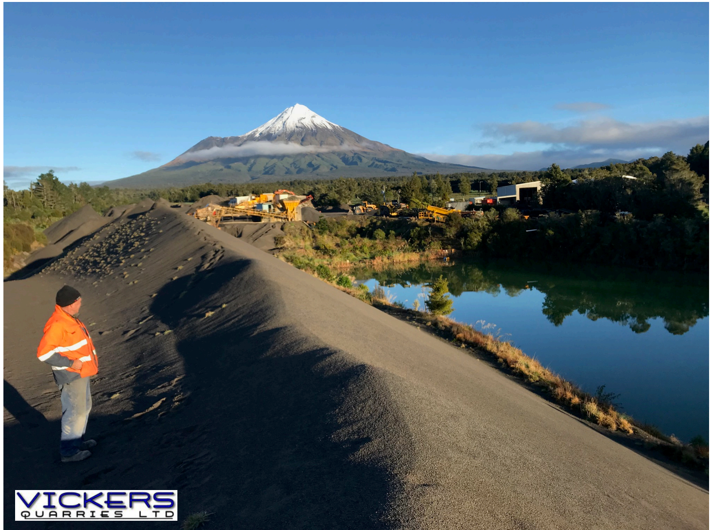
Bund around settling pond
