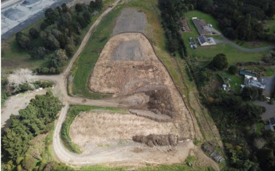
Figure 42: Construction of the noise bund in 2019.
