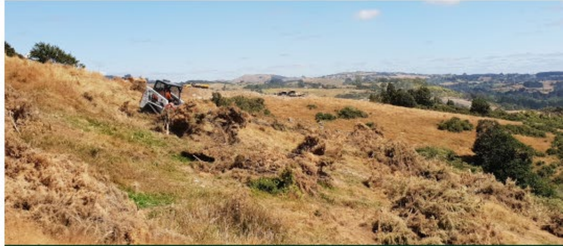
Figure 47: Use of a bobcat to stockpile removed noxious vegetation.
