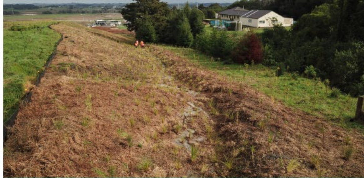
Figure 43: Swale on the eastern edge of the noise bund being planted with low growing wet-tolerant native species.
